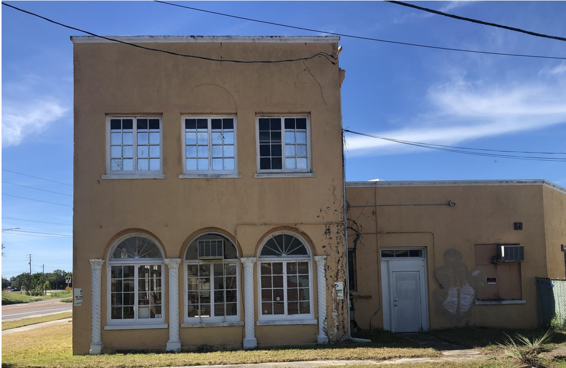
Northeast Facade - October 2021
