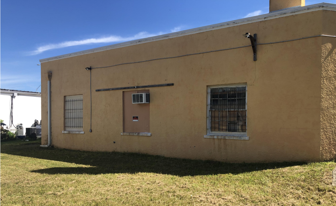
West Facade - October 2021
